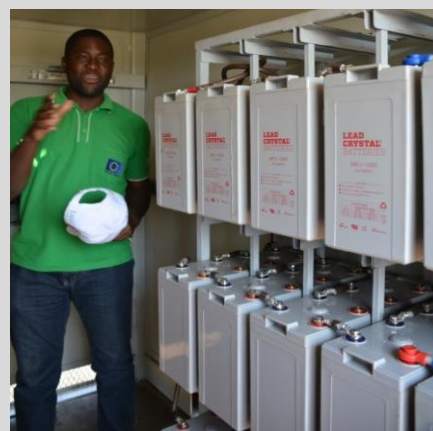
Figure 3: Mashaba clinic and mini-grid battery bank
